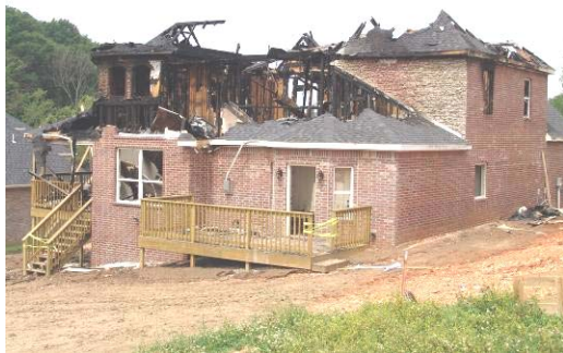
Figure 5: Destruction from inadequate ground
