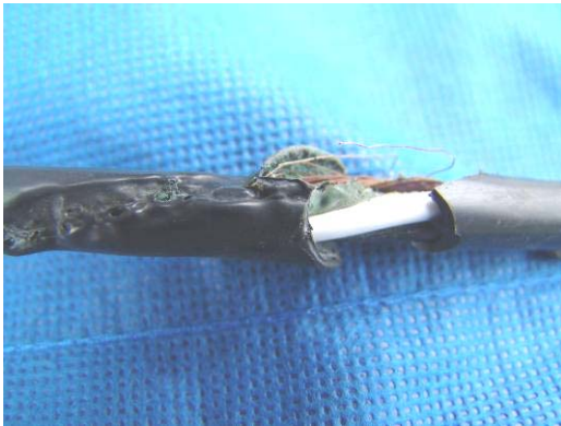
Figure 4: Ground conductor melted insulation
